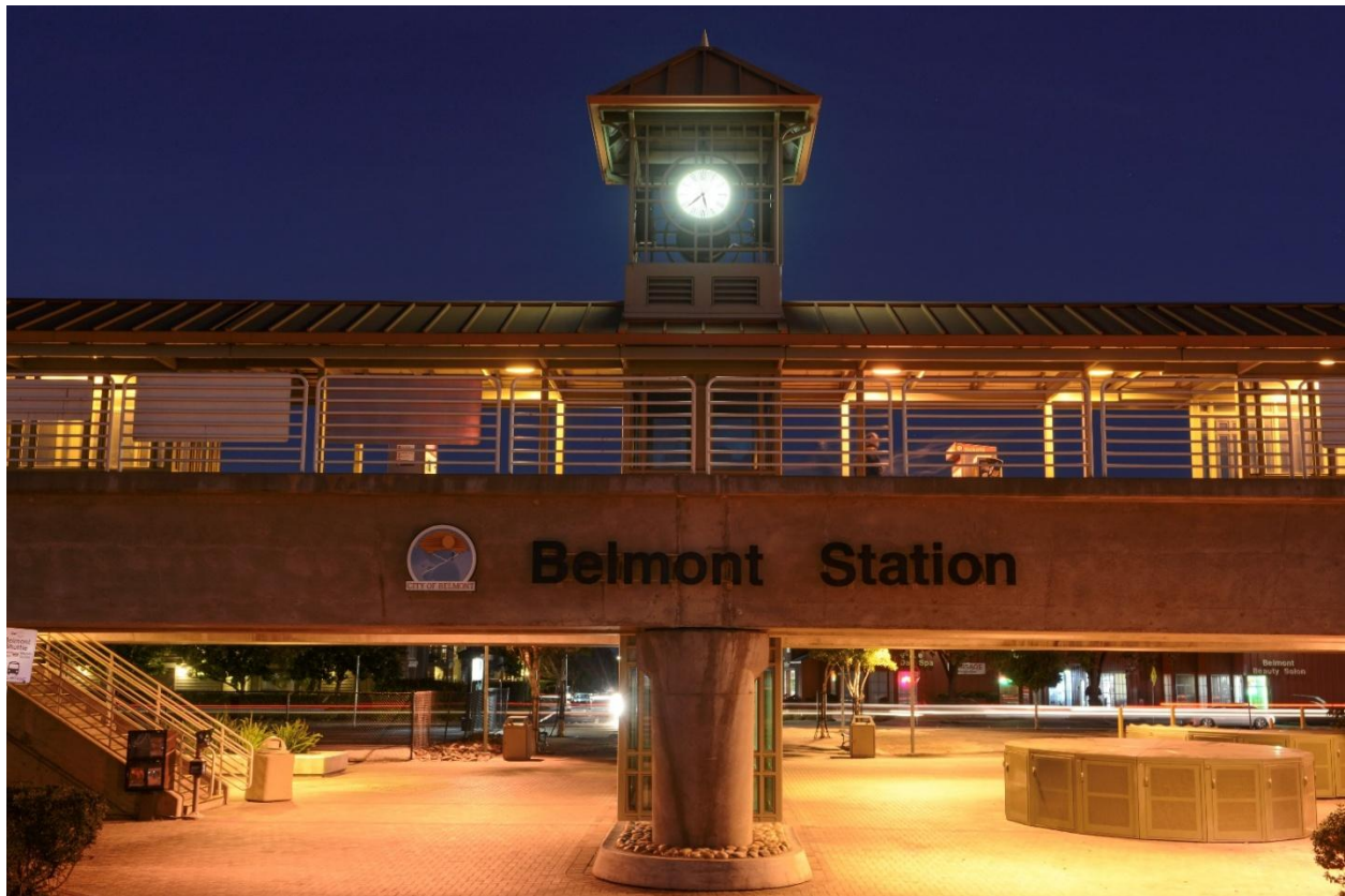
Belmont Caltrain Station. Source: City of Belmont
