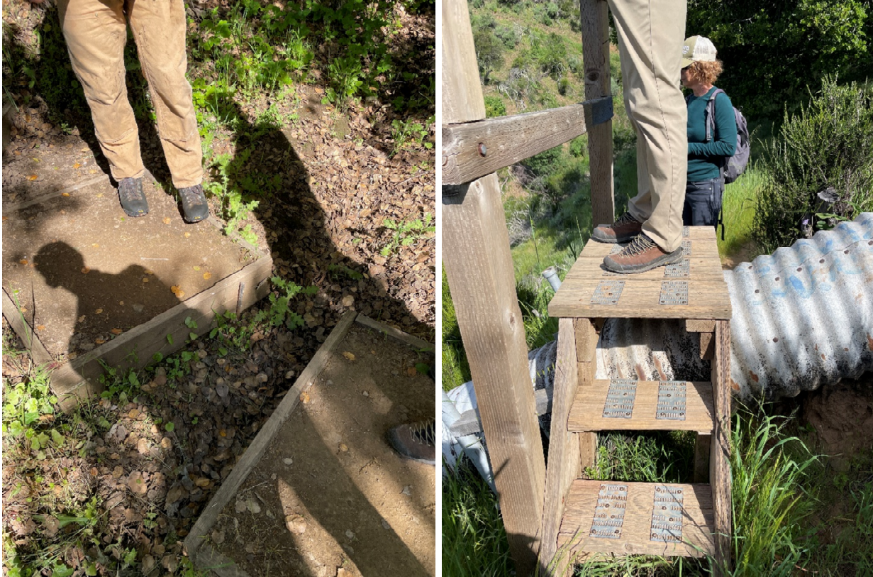
Left: example of existing stream crossing. Right: steps over drain pipe.
