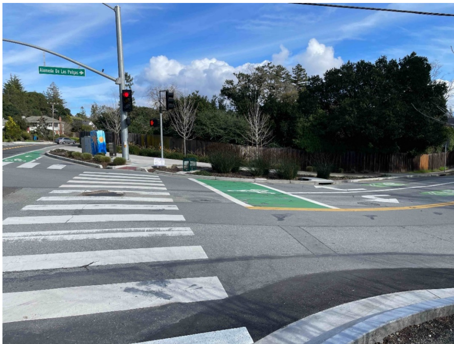
One of two LID treatments at San Carlos Ave and Alameda de las Pulgas with bike and pedestrian infrastructure.
