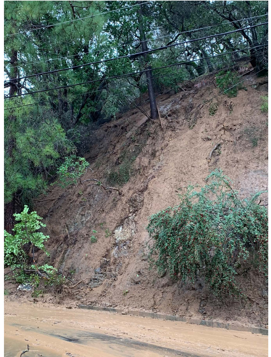
Figure 3.4 Landslide at Appian Way
