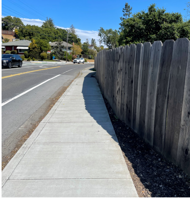
Fencing along San Carlos Ave sidewalk
