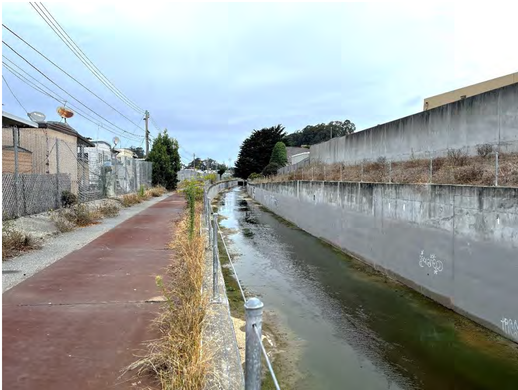
Photos 33 & 34 — Top and bottom photos show Colma Creek looking upstream toward the Mission Road Box Culvert.
