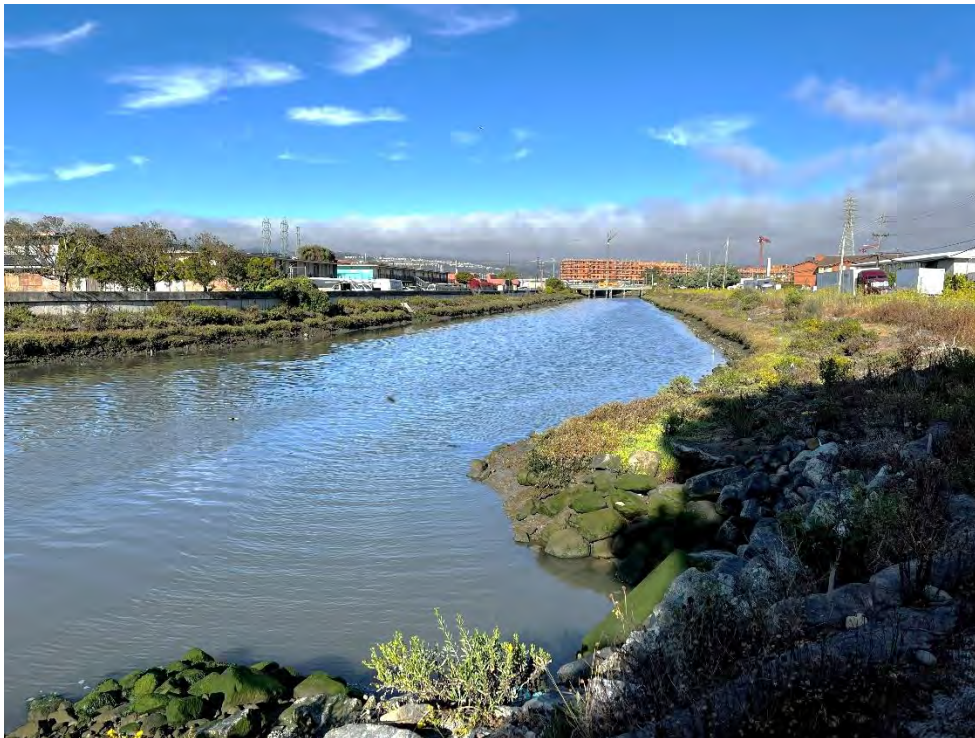
Photos 7 & 8 — Top photo shows Colma Creek looking downstream towards the Utah Avenue Bridge. Bottom photo shows Colma Creek looking upstream towards the S Airport Blvd Bridge.
